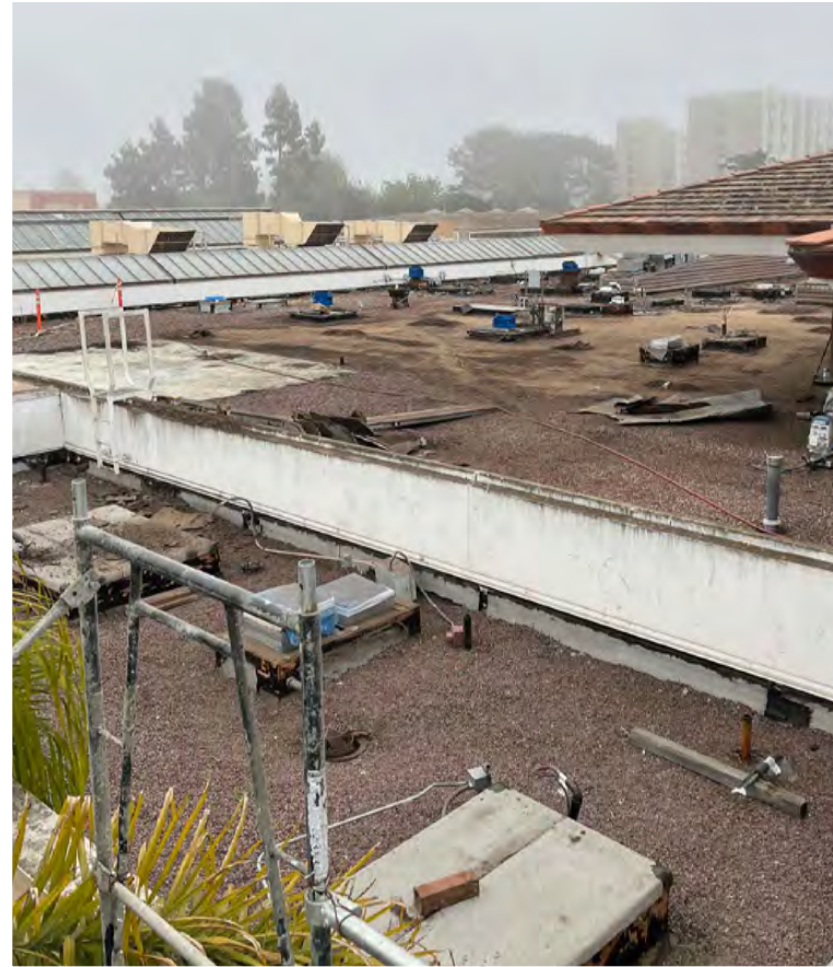
Photo of the University Center roof before the replacement and repair.
